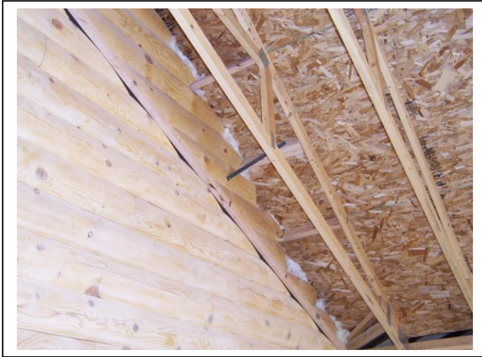
Figure 15. Unfinished cathedral ceiling showing trusses, log wall gabel and roof underlay.
