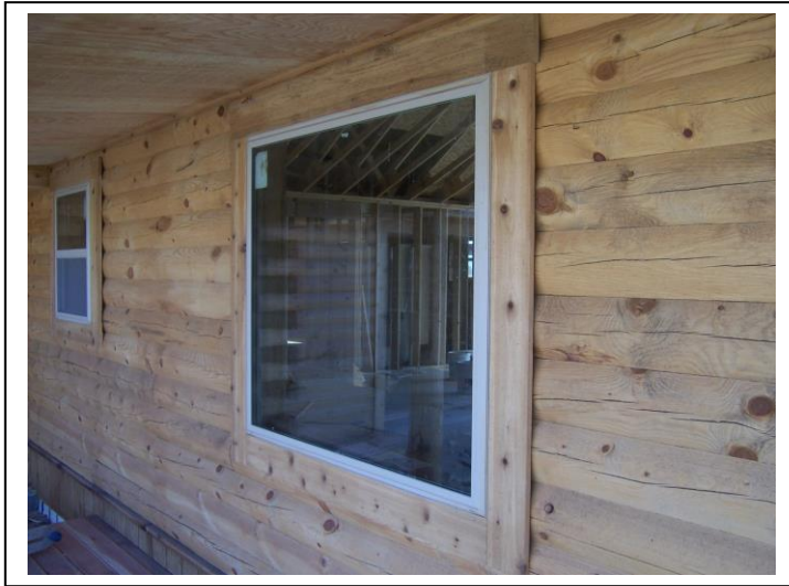
Figure 14. Completed window with trim.
