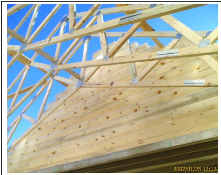
Figure 10. Gable log ends with trusses being installed for a cathedral ceiling.
