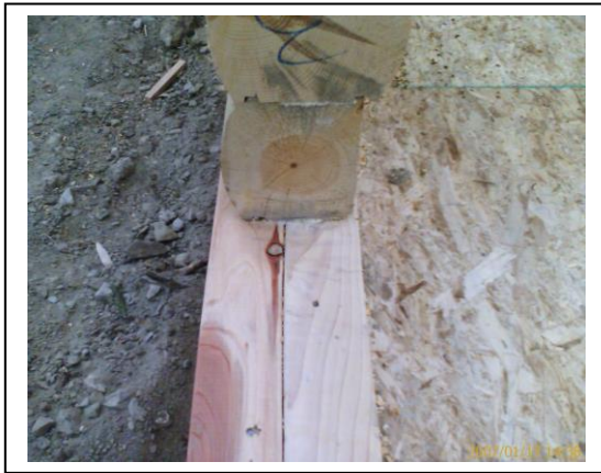
Figure 7. Properly installed drip ledge from another perspective.
