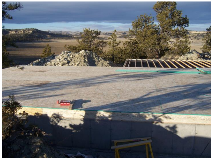
Figure 3 An almost completed sub-floor, soon to be ready for setting logs.
